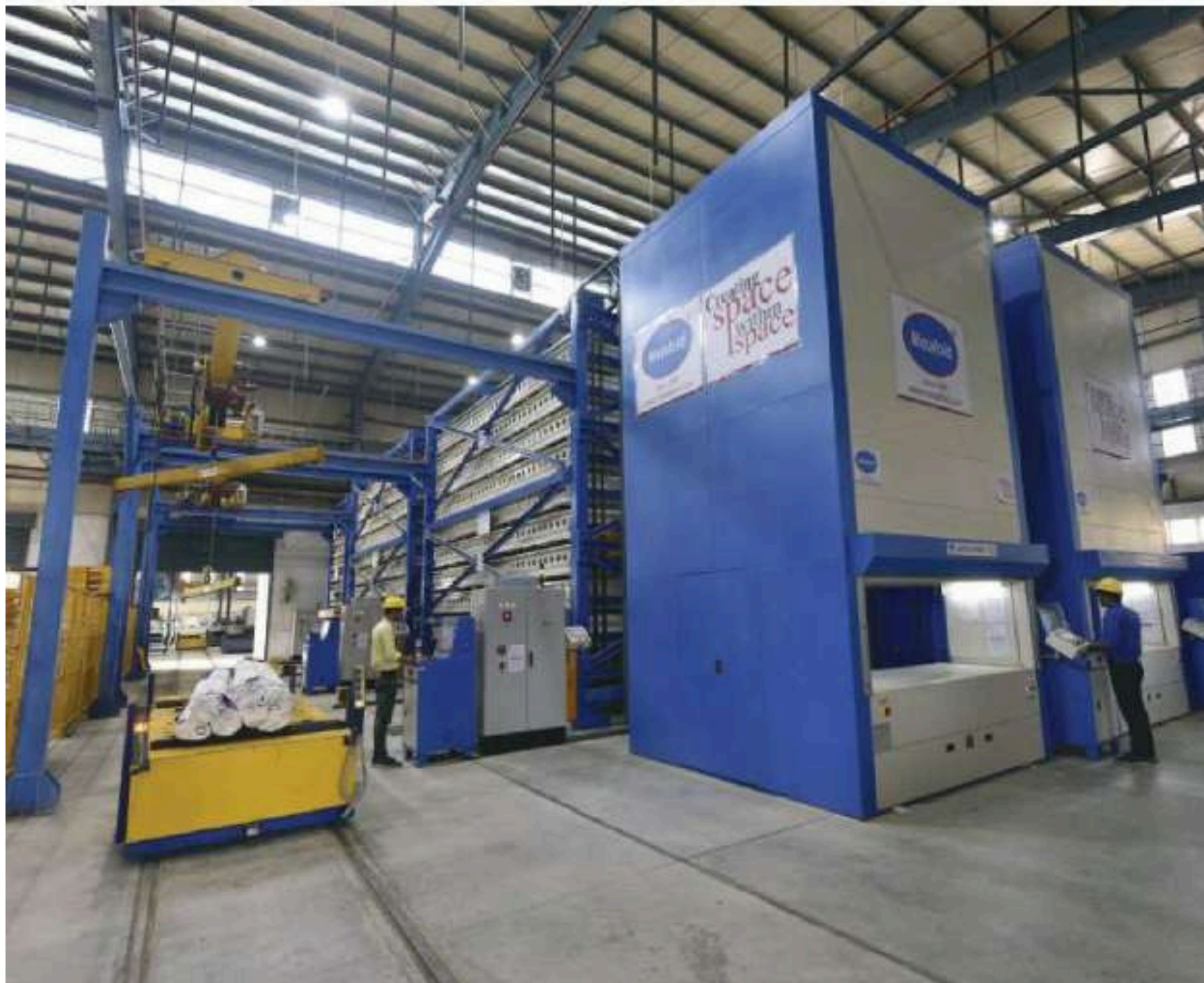
Automatic vertical storage SRAS system (Inside view of the Store)
