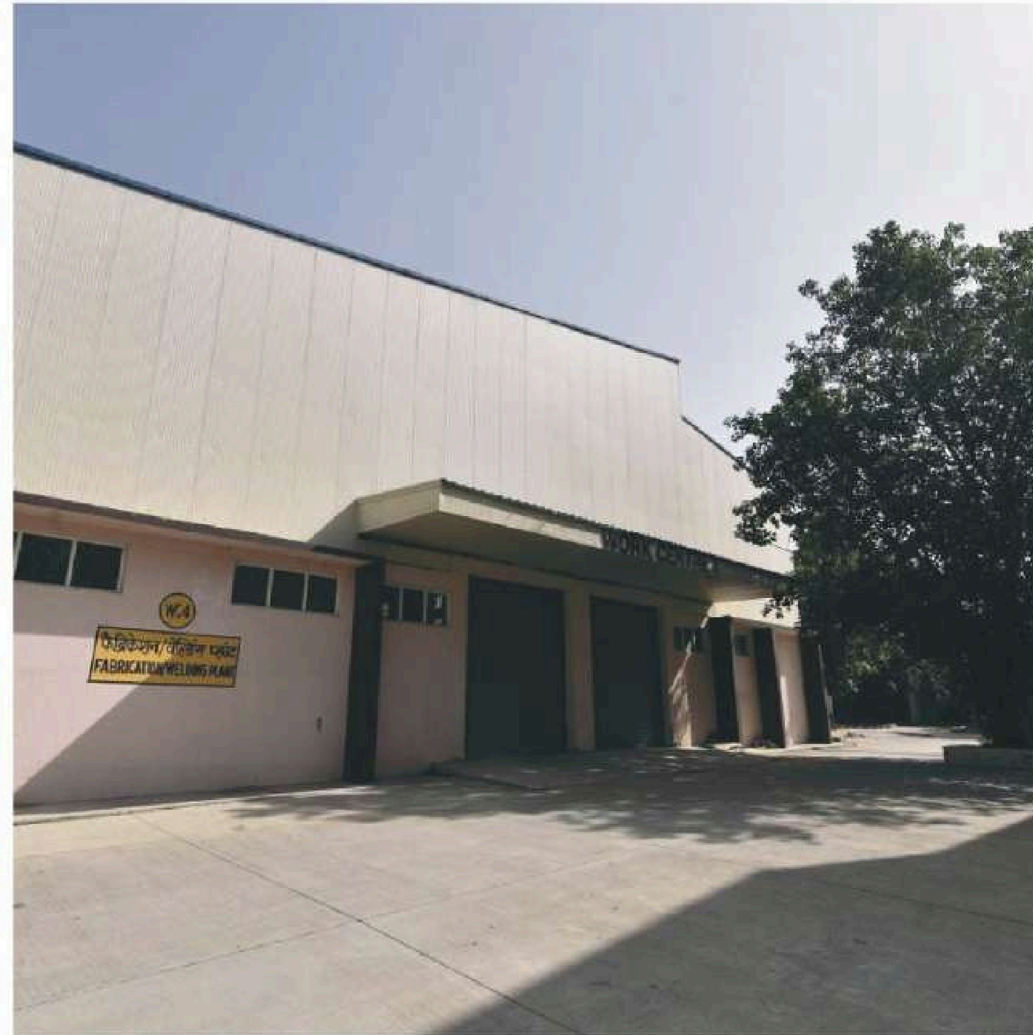
Robotic Welding Shop (work centre 4) :
